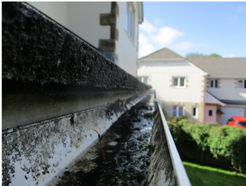
Front elevation gutter debris
