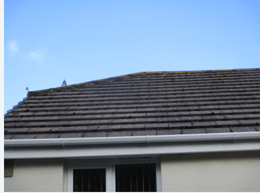
Rear elevation roofline
