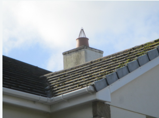
Front elevation roof valley
