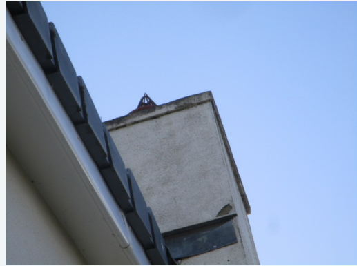
East elevation chimney stack
