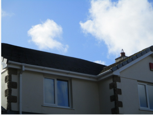
Front elevation roofline
