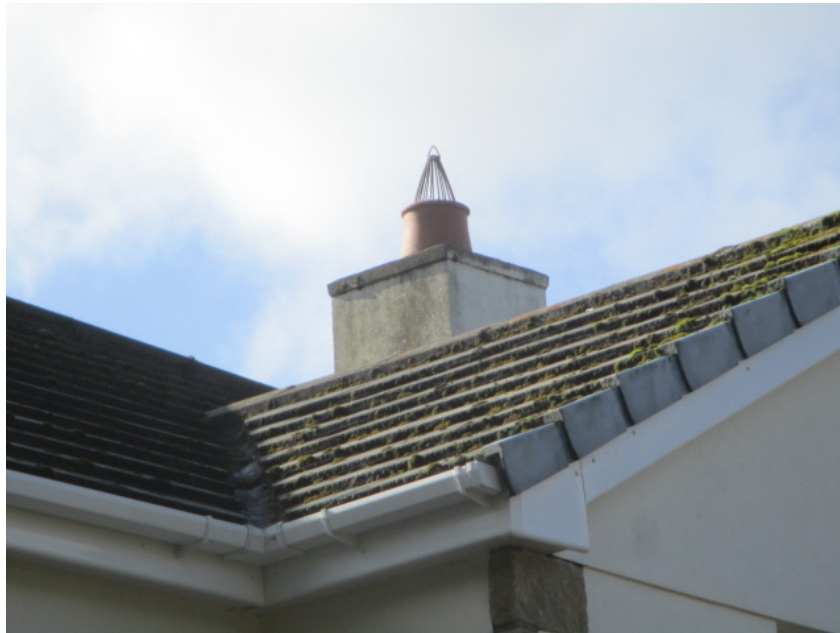
Front elevation gutter debris
